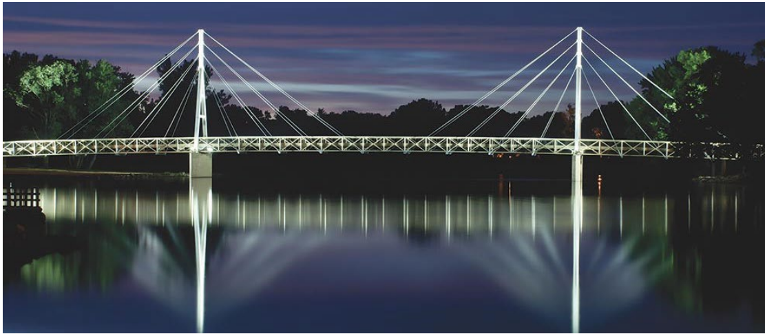
Figure 11. Example of a cable-stayed bridge
